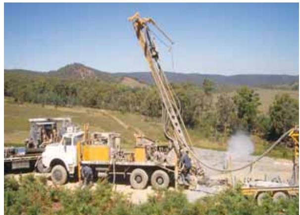
March 2008, Reedy Creek drilling
