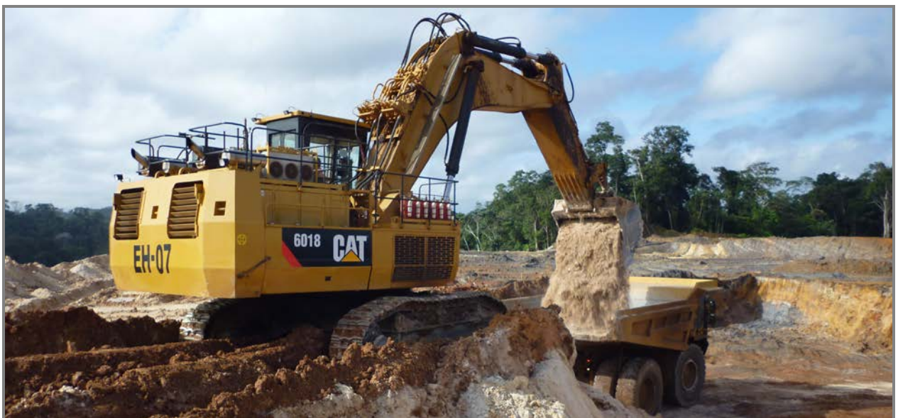
Photo 2. Cat 6018 excavator loading trucks at newly established Urucum Pit
