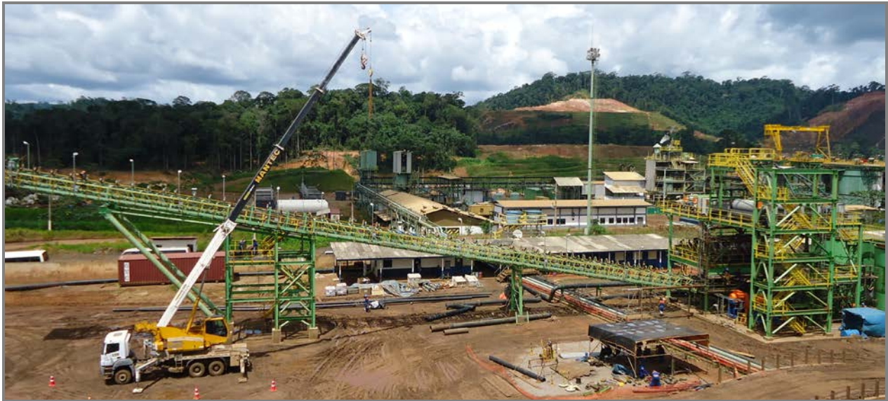
Photo 1. Iron Ore Concentrate Plant nearing completion
