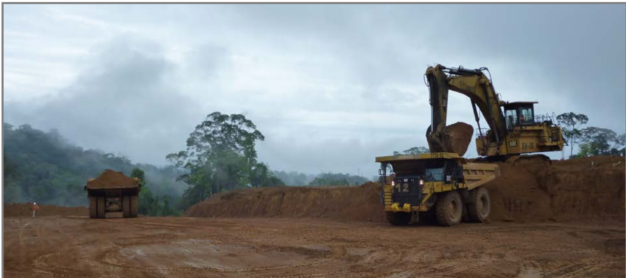
Photo 1. Mining commenced at the ultra high grade Duckhead gold deposit
