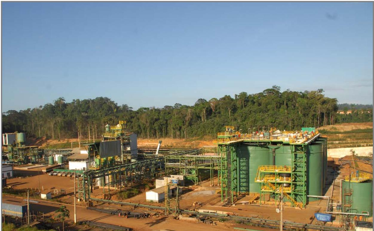
Photo 1. Completed CIL plant including gold elution circuit
