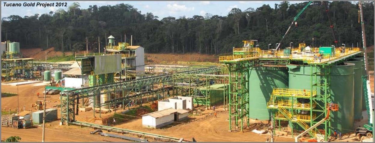
Photo 1. CIL Tanks, Gold Room and Elution circuit nearing completion
