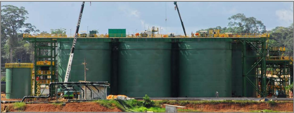
Photo 2. CIL Tanks and Top of Tank Steel completed
