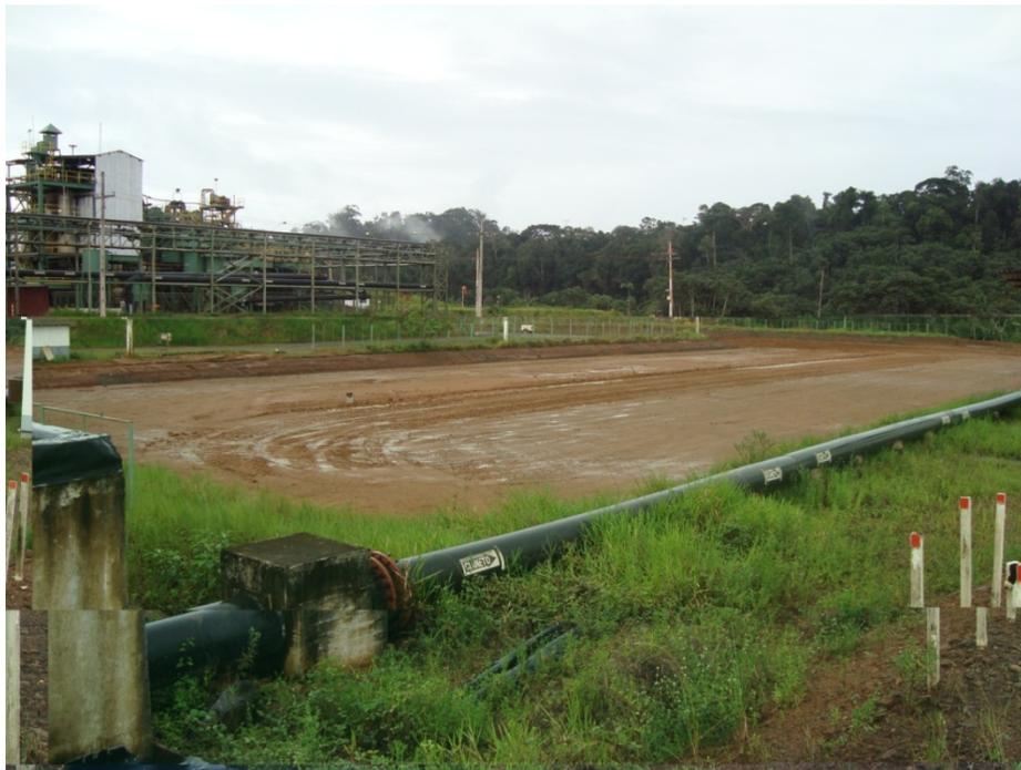
**Pregnant liquor pond backfilled and ready for CIL tanks**
