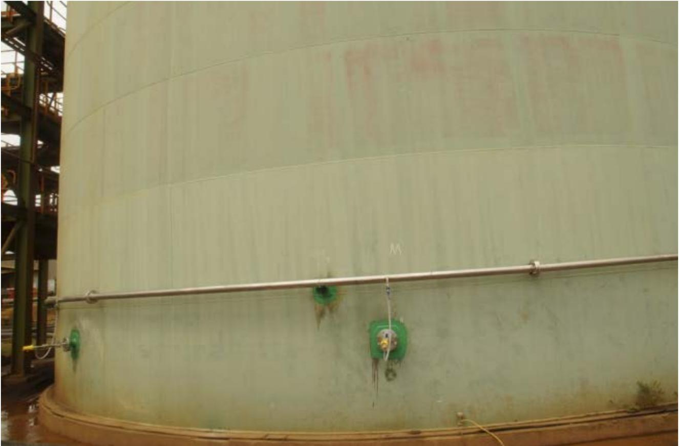
Photo 6: Tank 1 external sparger housing.
