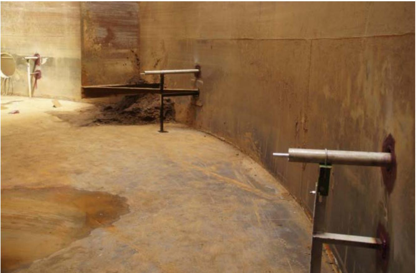
Photo 5: Tank 1 internal sparger configuration
