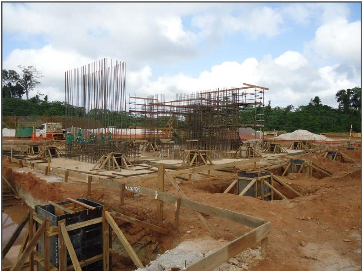
**Photo 2 - SAG mill foundation poured – plinth rebar being prepared.**
