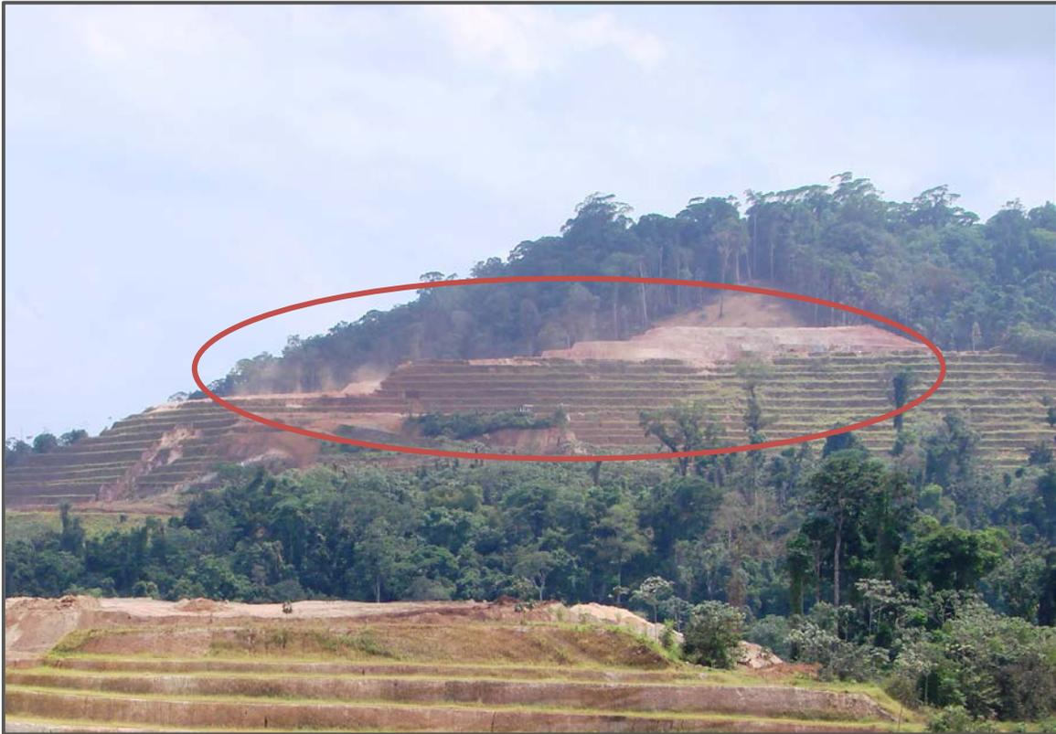
**Photo 5 – Tap AB2 eastern wall in the background showing clearing and cutback in progress**
