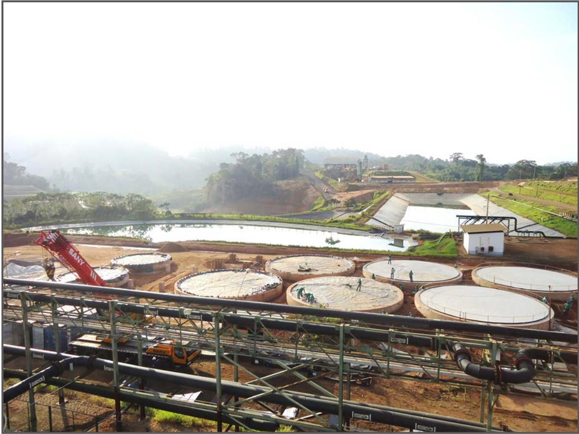
**Photo 1 – CIL and cyanide detox tank rings being prepared for tank steel (tank steel being unloaded in the foreground)**
