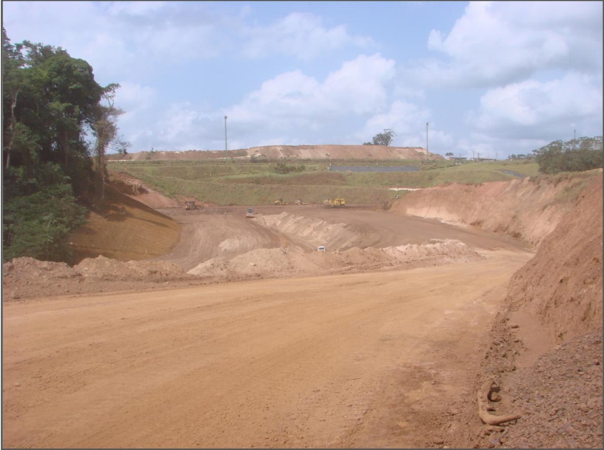
**Photo 7 – Tap D tailings dam under construction with the new ROM in the background**
